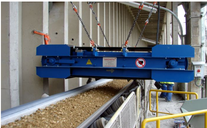
Removal of tramp iron from clinker.
