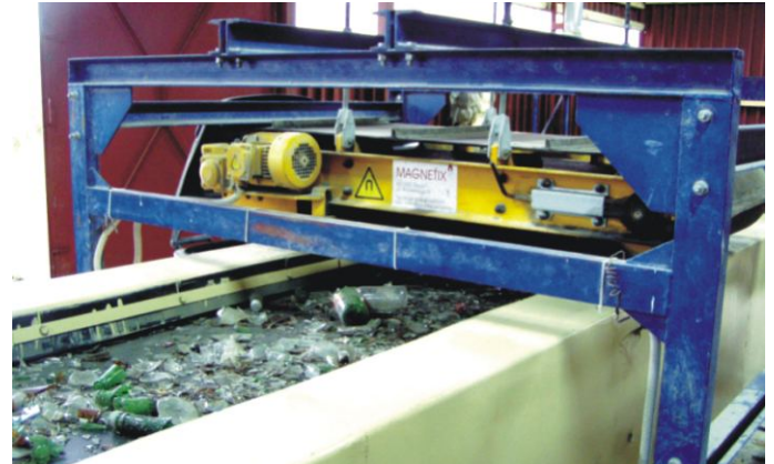
Separation of ferrous scrap from glass cullet.
