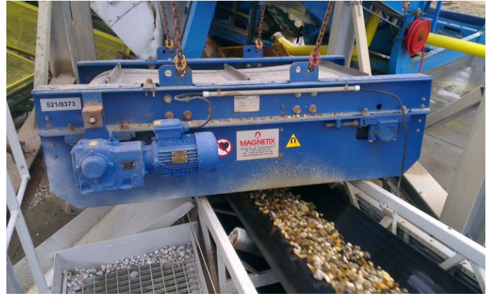
Removal of tramp iron contaminants from gravel.
