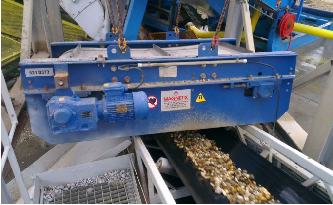
Removal of tramp iron contaminants from gravel.
